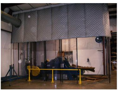
Ceiling mounted track systems allow for panels to easily slide past one another for superior access.
