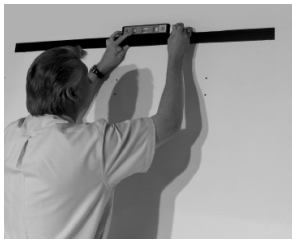
Step 1: Use level to mark top line. Step 2: Repeat for set line.
