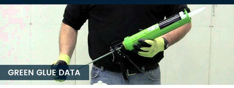
Green Glue is a liquid, waterborne, viscoelastic damping compound which represents the highest performance product of its type. It is used in between sheets of drywall, subflooring or other building materials. It is significantly lower in applied cost than competitive products, with an excellent cost/performance ratio. It is also remarkably tolerant to real-world application conditions and carries almost none of the burden of precision required by many damping systems.
