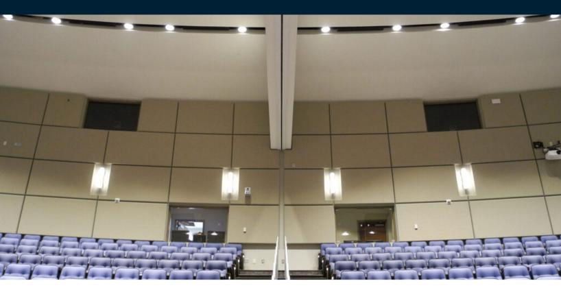
Acoustical Wall panels are sound absorbing panels that can mount directly to walls or ceilings through a variety of adhesives, impaling clips, hook & loop fasters etc. They are designed to stop noise control issues with their powerful sound absorbing acoustical materials. They are frequently used in offices as they not only prevent noise pollution but increase speech intelligibility by reducing reverberation and echoes
