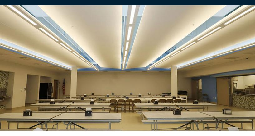
Ceiling Clouds are perfect for the reduction of sound in ceiling areas. They are suspended horizontally with D-Ring (for panels up to 4' x 4') or T-grid attachment for larger panels
