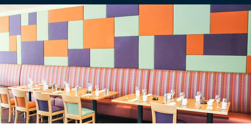
Acoustical Wall panels are sound absorbing panels that can mount directly to walls or ceilings through a variety of adhesives, impaling clips, hook & loop fasters etc. They are designed to stop noise control issues with their powerful sound absorbing acoustical materials. They are frequently used in offices as they not only prevent noise pollution but increase speech intelligibility by reducing reverberation and echoes
