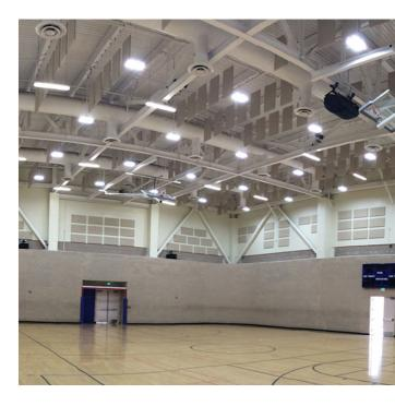
The panels are installed approx 30" apart over the entire reverberant area and can result in an astounding 4 to 12 decibel reduction in general noise.
